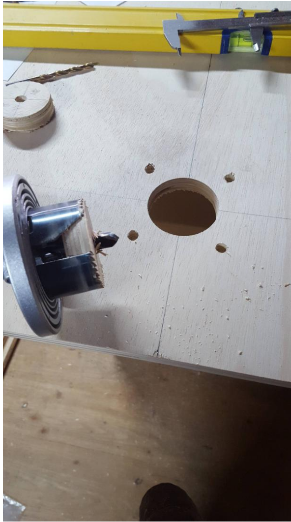
Figure 2.8. Holes drilled out
